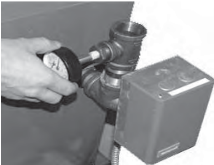
Figure 8 - Thread Gauge Into Supply Water Tee
